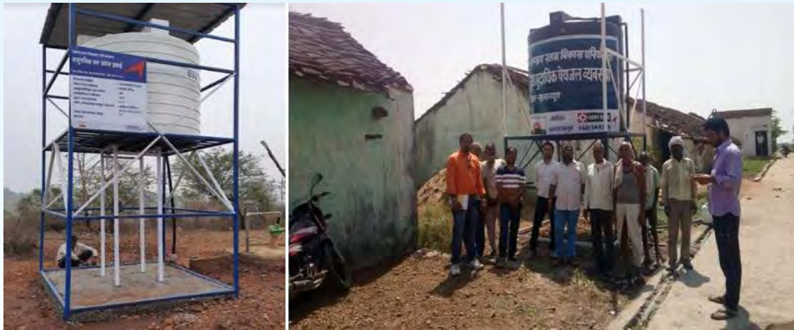
Figure 6: Overhead tank installed; construction work in progress
